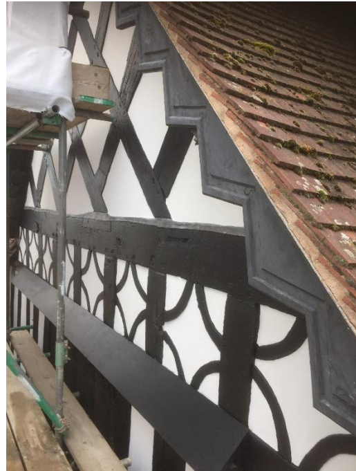
Pic. East gable completed
