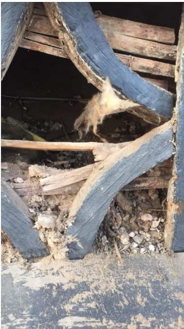
Pic. East gable before works
