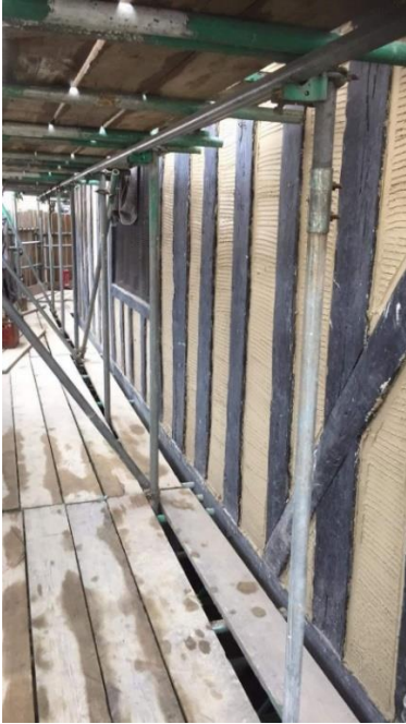
Pic. First coat of lime render
