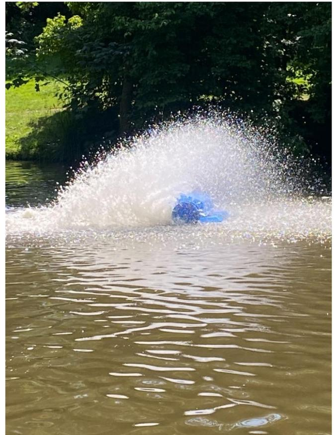
Pictured above is the new aerator at the Lake, which is switched on during hot weather, to maintain oxygen levels. This aerator was obtained using Environment Agency funding.
