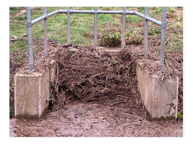
It is also proven not to work as the screen has frequently not been cleared by FODDC at times of rainfall. In this case if the screen is not cleared prior to rainfall then operatives are unable to reach the screen because of increasing water levels.
